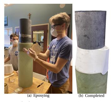
Figure 14: Payload Bay Construction: Epoxying Transition Section
