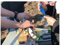
Figure 114: Z-Fold of Shock Cord and Application of Painter's Tape
