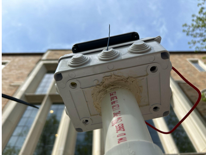
Figure 8. Enclosure with Ventilation
