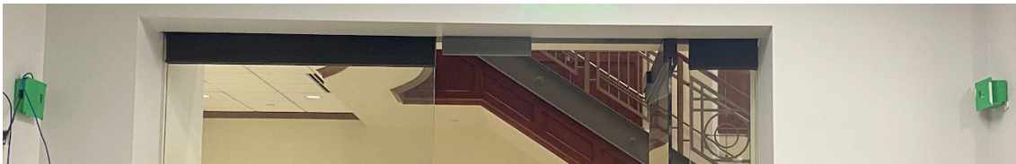
Figure 13. Example Setup of Transmitter and Receiver Modules
